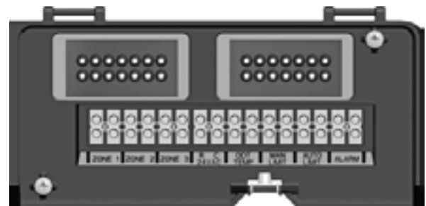
Low voltage wiring terminals
